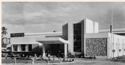
— The Rane (Madras) Limited administrative block at Velachery, reflecting the company's expanding manufacturing presence.
